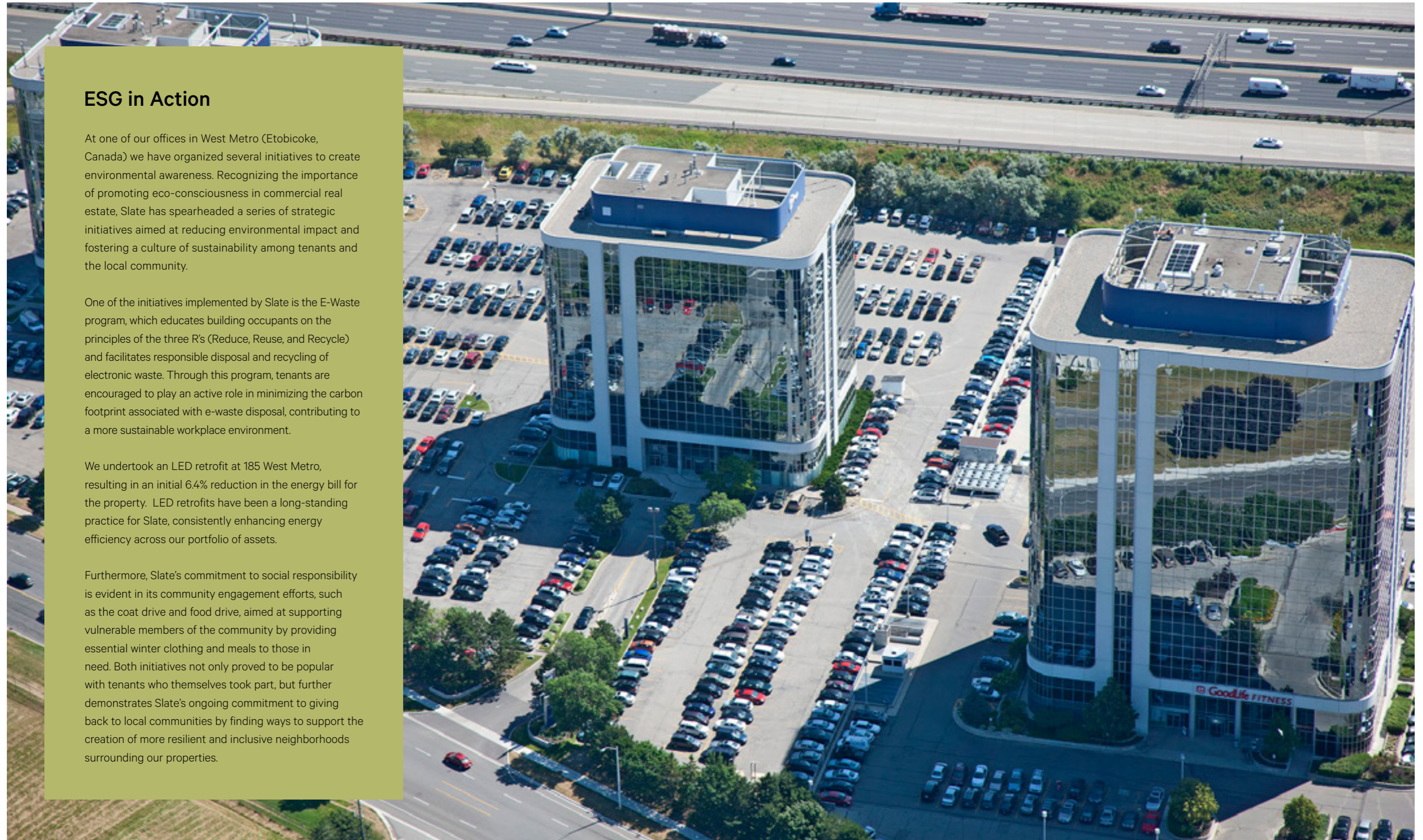
West Metro Corporate Centre, Ontario, Canada
